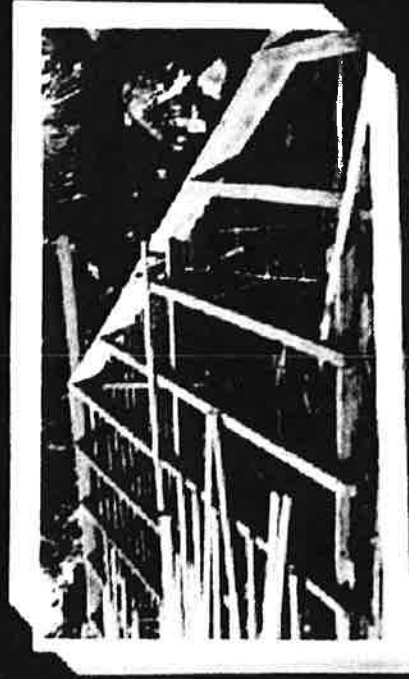
ii. do the roof construction here, number each piece, take the roof apart and haul it to the Paul Islands, to build Schools and Churches.
